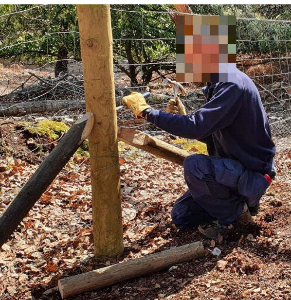
Below: Learning to install fencing
