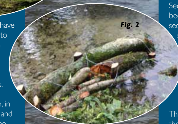
'Berm' created on Sydling Water to change the flow
